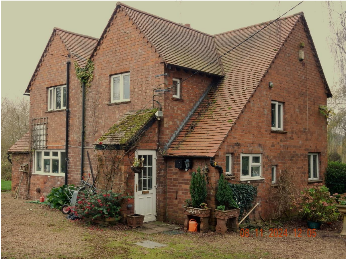
The photograph shows Debden Cottages as they are at November 2024. Number 1 was the nearer part of the building but the two cottages have now been combined into one dwelling.
